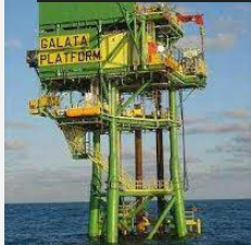
GTP and Offshore jacket
