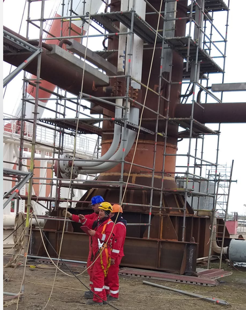
Construction and commissioning of Oil & Gas rigs
