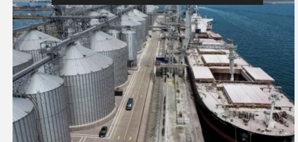
Port operation terminal
